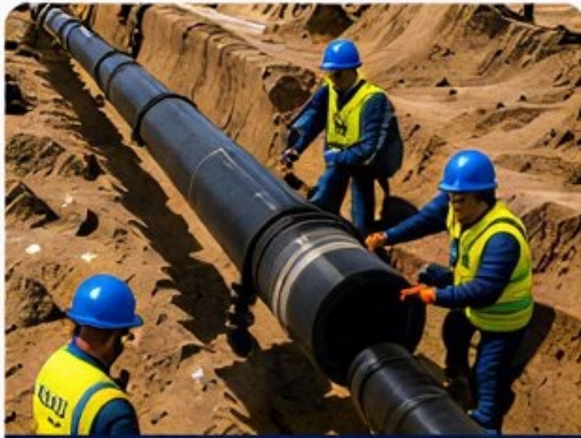
SEWAGE PIPELINE NETWORK PROJECT
