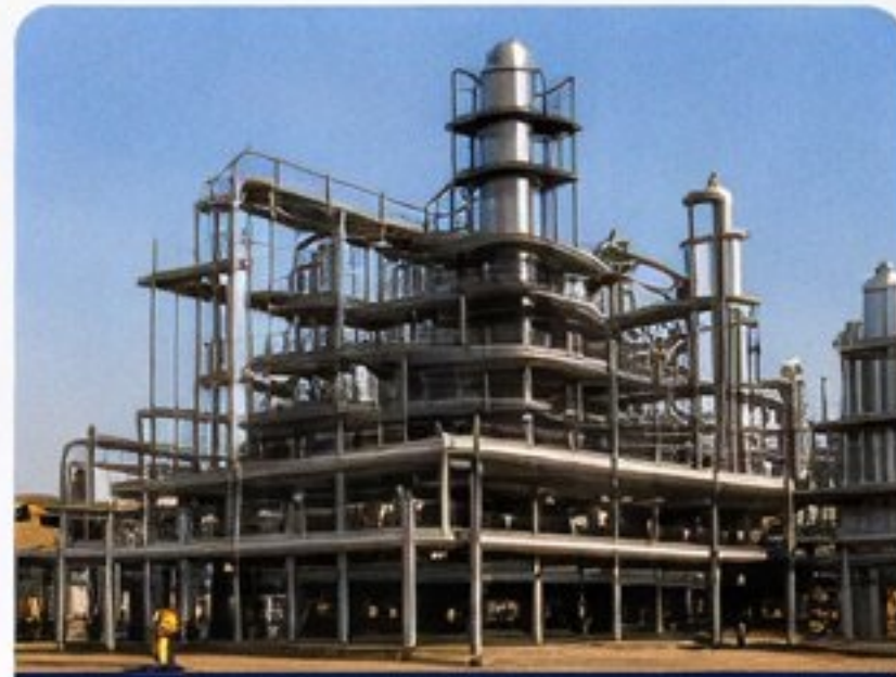
INDUSTRIAL PIPELINE INSTALLATION
