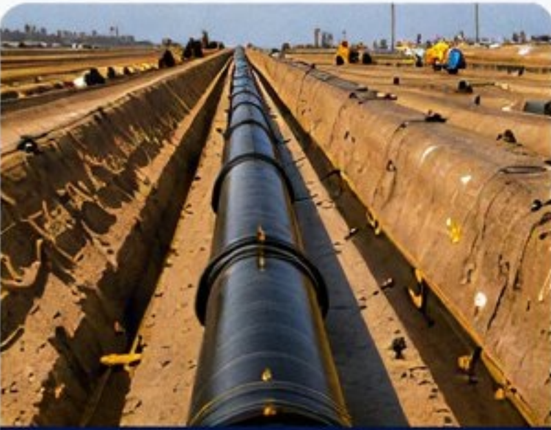
HDPE WATER PIPELINE INSTALLATION
